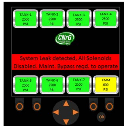
Figure 96. System Leak. Maintenance Bypass Required.
