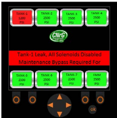
Figure 94. Tank 1 Leak. Maintenance Bypass Required.
